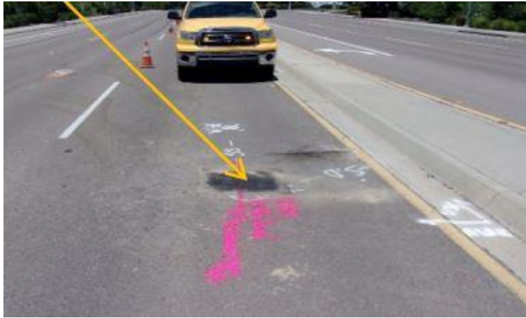
Figure 4: Potholing Location After Restoration
