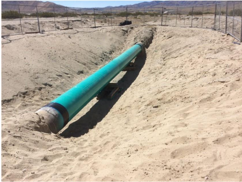
Figure 11: Pipeline Excavation and Repair Site
