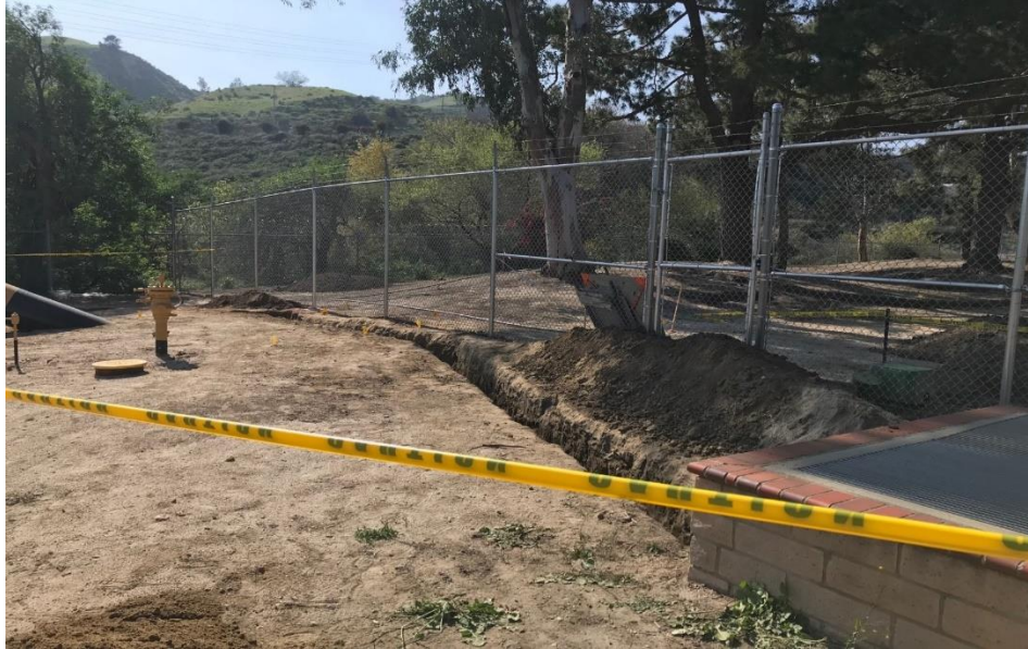
Figure 10: Hand Dug Trench
