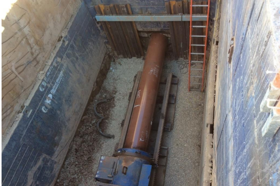
Figure 27: Boring Machine Pushing Casing Pipe
