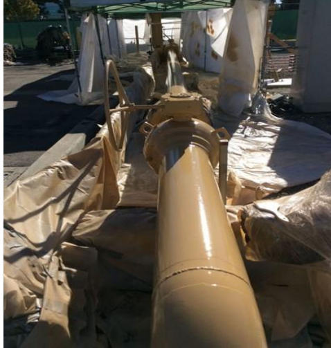
Figure 23: Electronic Inspection method - Holiday Testing of a Coated and Wrapped Weld
