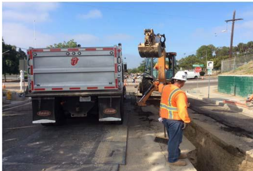
Figure 8: Trench Excavation with Backhoe
