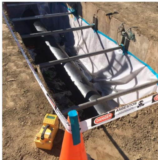
Figure 5: Typical Pipeline Abatement
