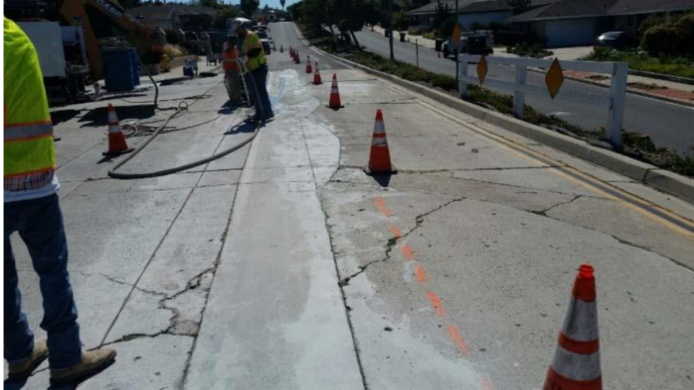
Figure 7: Saw Cutting Trench Pathway
