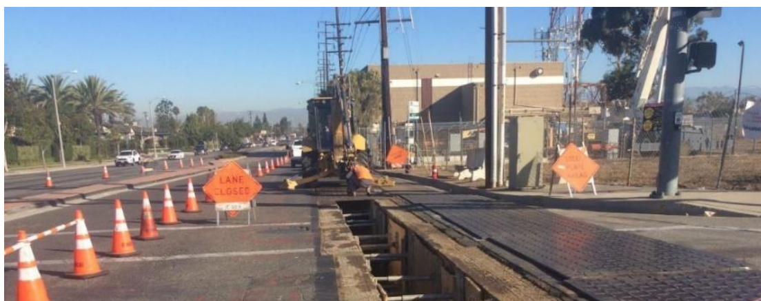
Figure 1: Traffic Control Lane Closure
