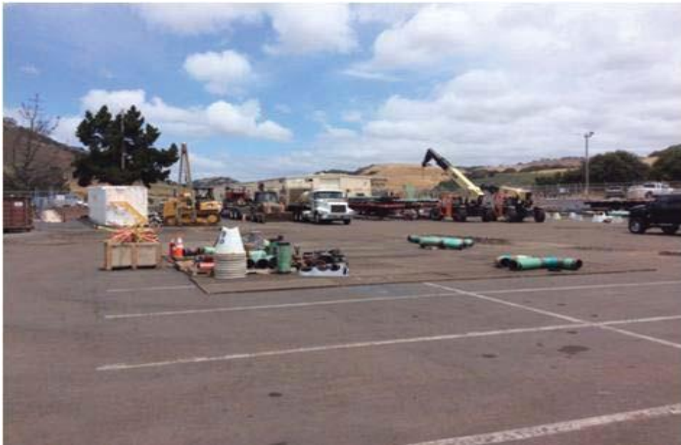
Figure 6: Construction Laydown Yard
