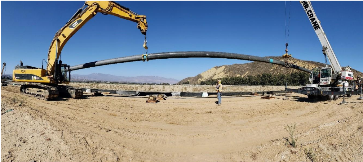
Figure 14: HDD Pullback
