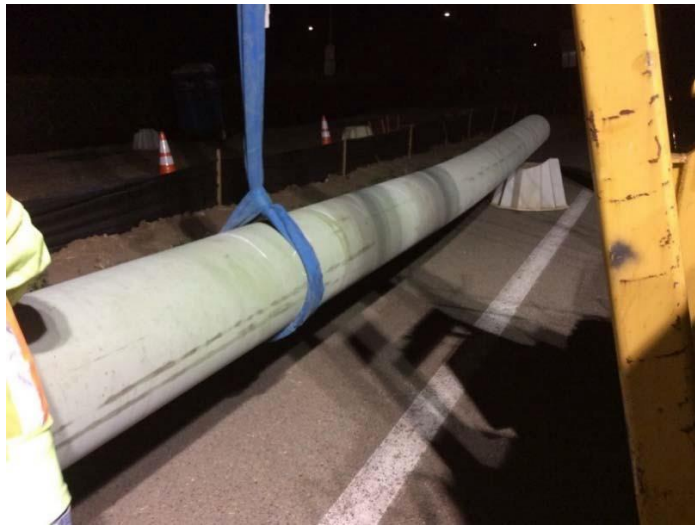
Figure 19: Pipe with Field Bend Laying on Supports
