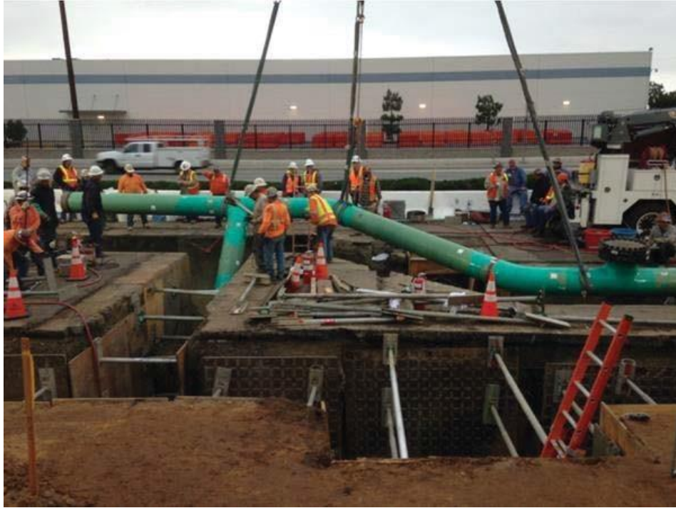
Figure 21: Lowering Section of Pipe into the Trench
