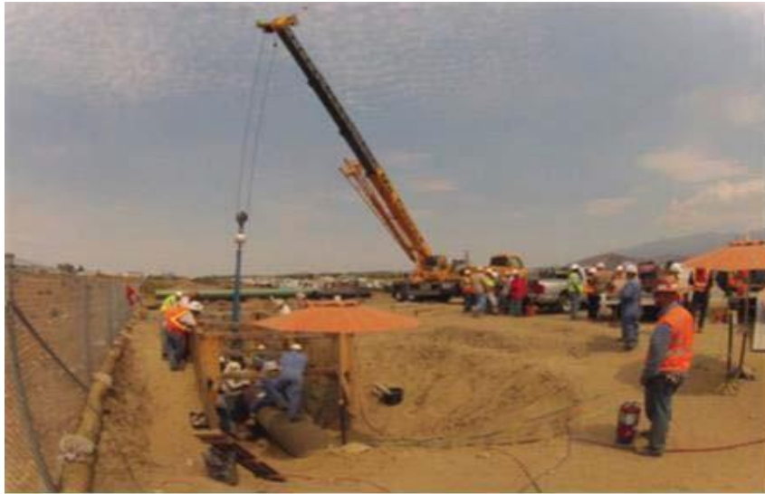
Figure 28: Checking for Leaks Before Start of Line Odorizing
