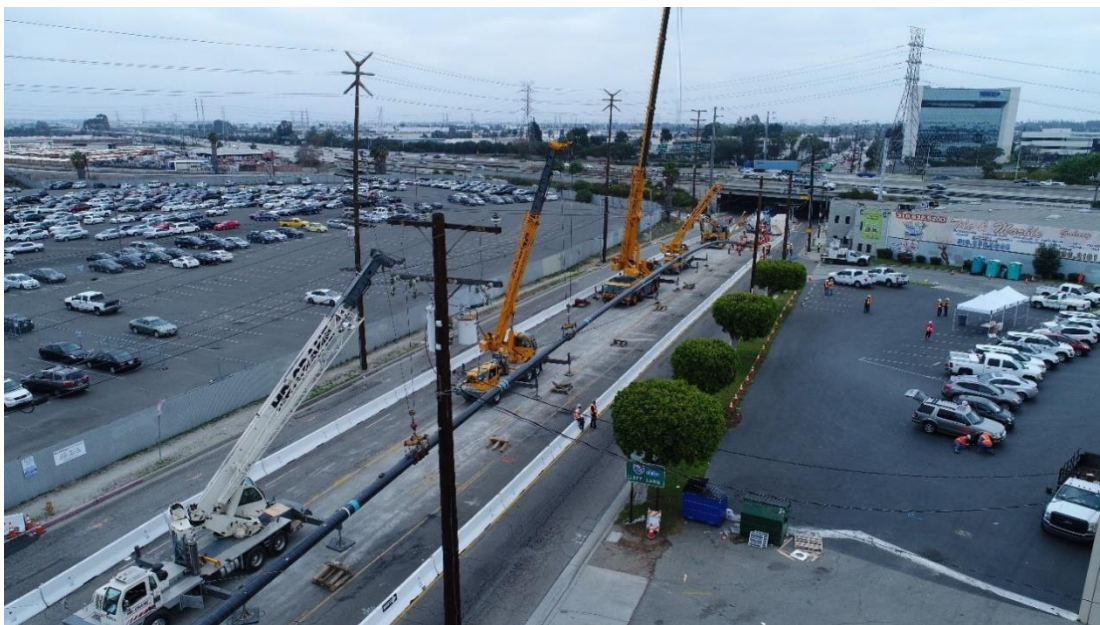
Figure 15: HDD Pullback
