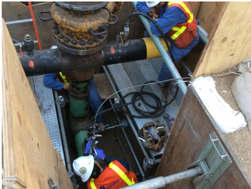
Figure 28: Checking for Leaks Before Start of Line Odorizing
